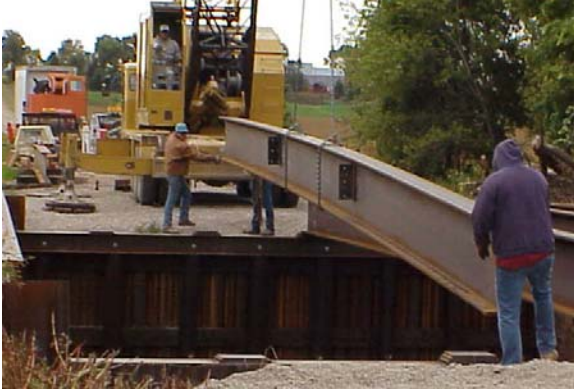
(a) Setting the girders into place
