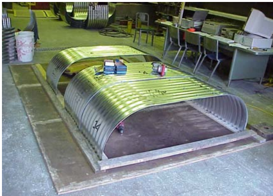
(c) Assembling the segments
