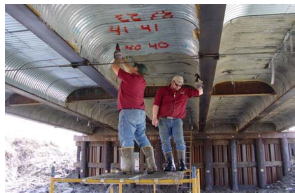
(b) Removing the arched formwork
