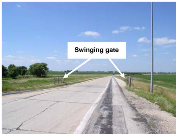
**Figure 4.1. Gates on entrance ramp to I-35**
