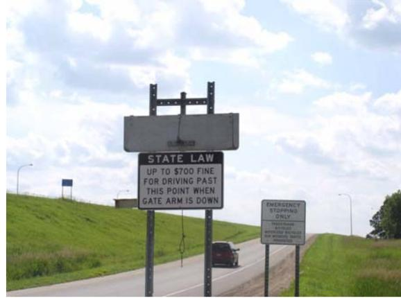
**Figure 1.4. Minnesota flip-down ramp closure sign**
