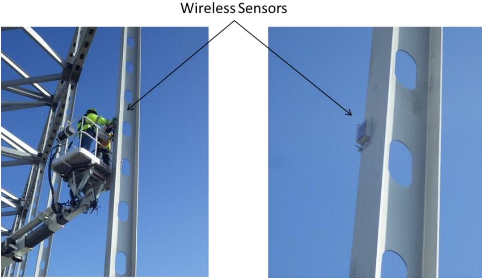
**Figure 13. Installation of wireless sensor nodes**
