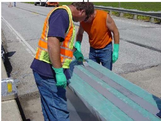
(c) Epoxy application on CFRP plates
