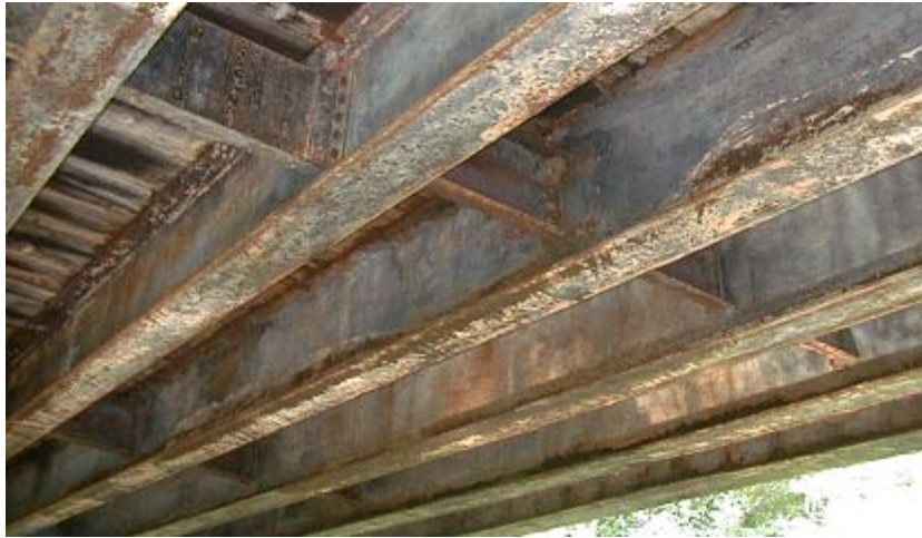
FIGURE 2. Photograph of Bridge Superstructure
