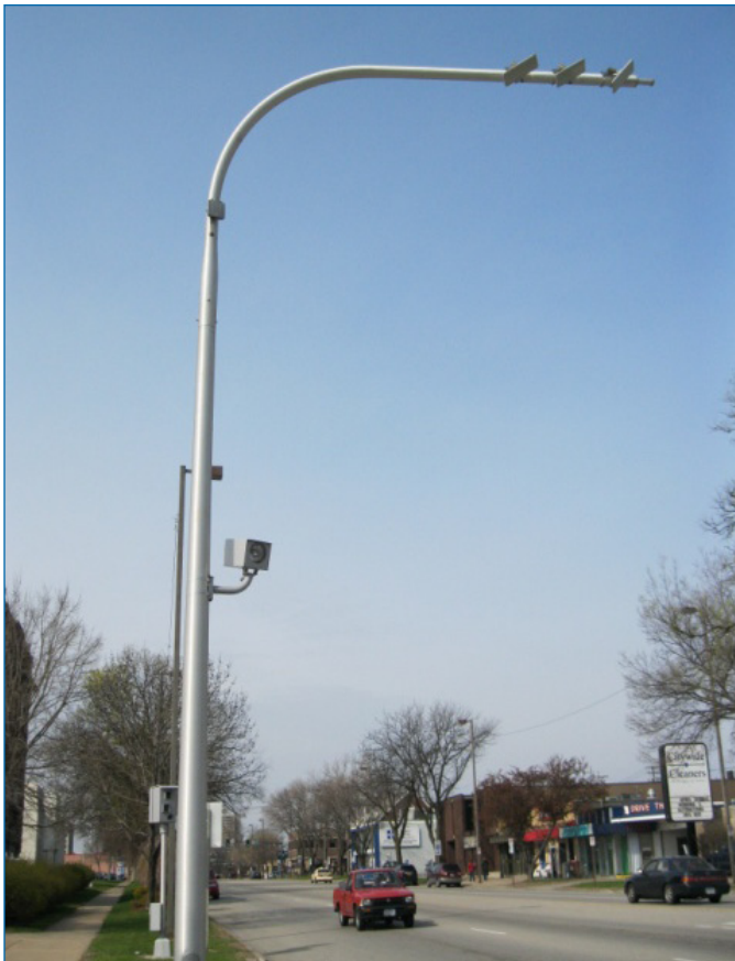
Mast arm and Radio Frequency antennae setup
