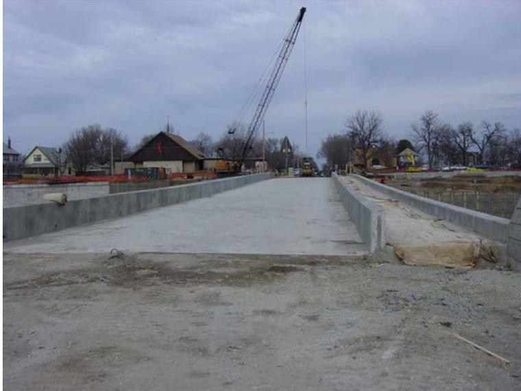
**Figure 3.26. Bridge after slip forming of barriers**
