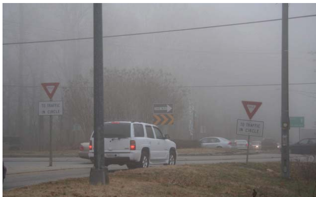
Unbalanced flow at roundabout
