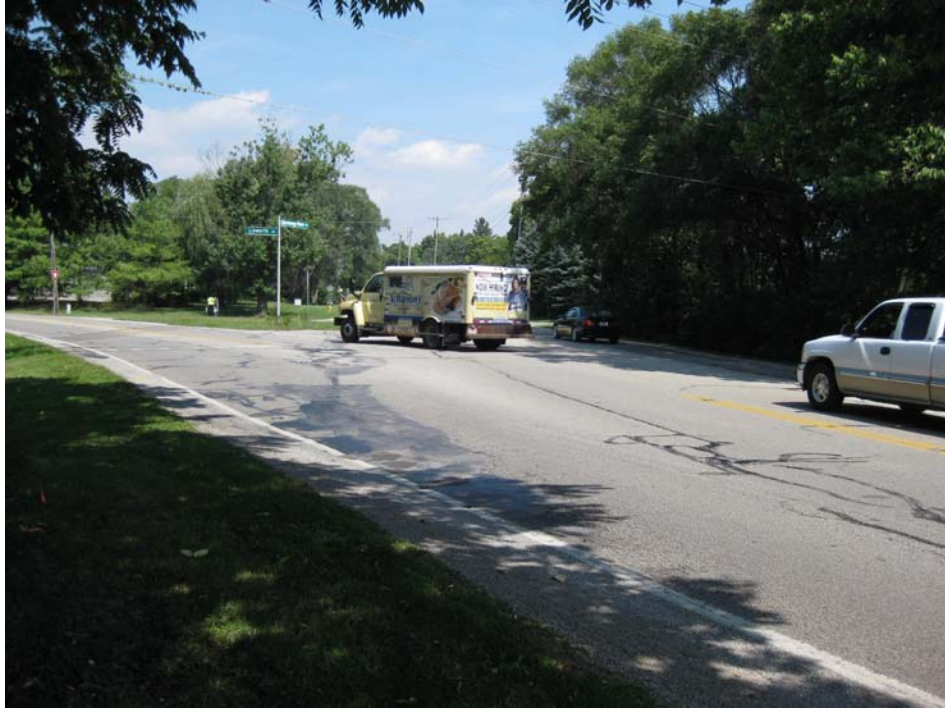
Figure A.6. Use of left-turn storage lane from northbound Olentangy River Road
