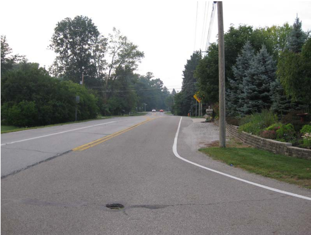
Figure A.4. Advance YIELD sign on southbound Linworth Road, hampered by vegetation
