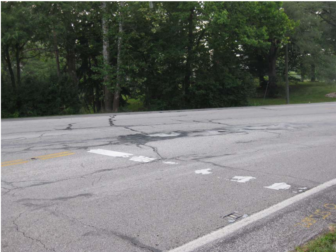
Figure A.5. Pavement markings on southbound Linworth Road
