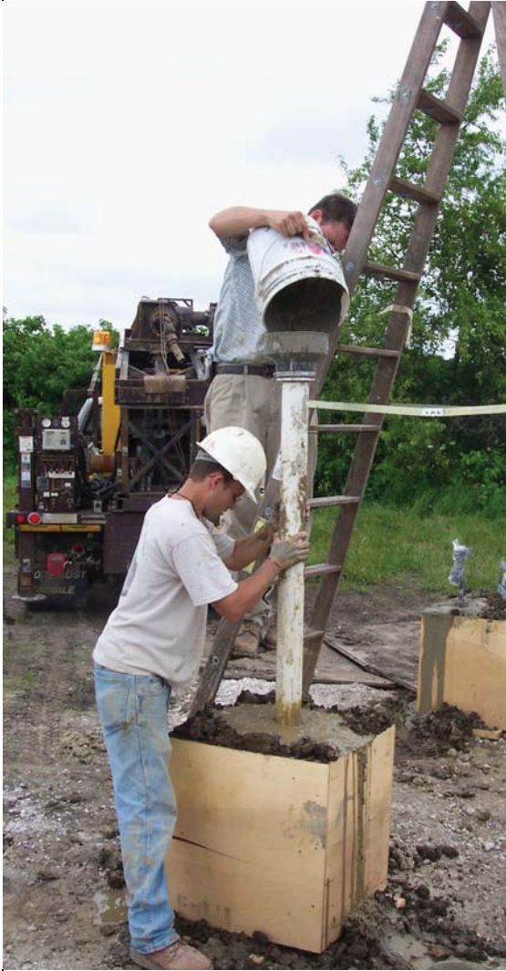
High-slump grout placement during pile installation for load tests
