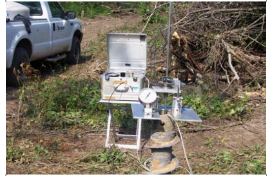
Iowa BST performance using hollow-stem auger as borehole casing
