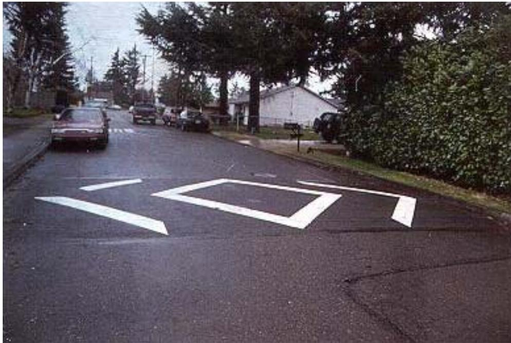
**Figure 1. Typical Speed Hump
