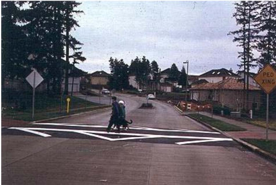
**Figure 2. Typical Speed Table
