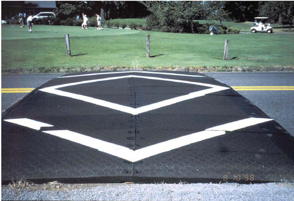
**Figure 17. 14-Foot Temporary 25 mph Speed Hump
