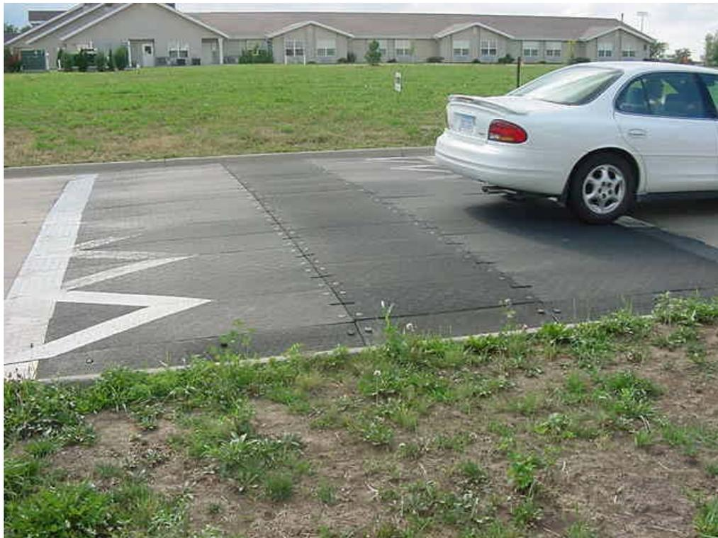
**Figure 18. 18-Foot Temporary 30 mph Speed Table**
