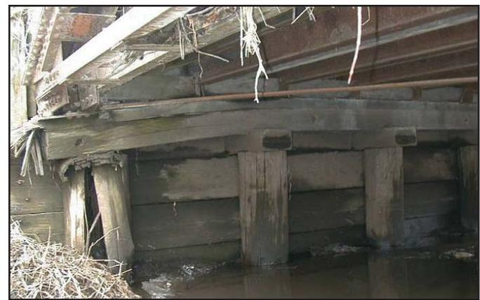
Biological deterioration resulting in reduction in pile cross section (top) and complete deterioration of a pile section causing failure of pile cap (bottom)
