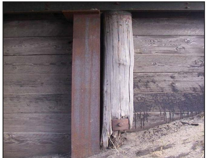
*Steel pile driven adjacent to a defective timber pile*
