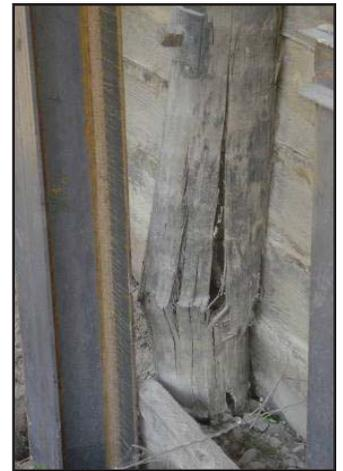
*Compression failure of deteriorated pile section caused by overloading leading to bulging of timber fibers (left) and mushrooming of the pile section (right)*
