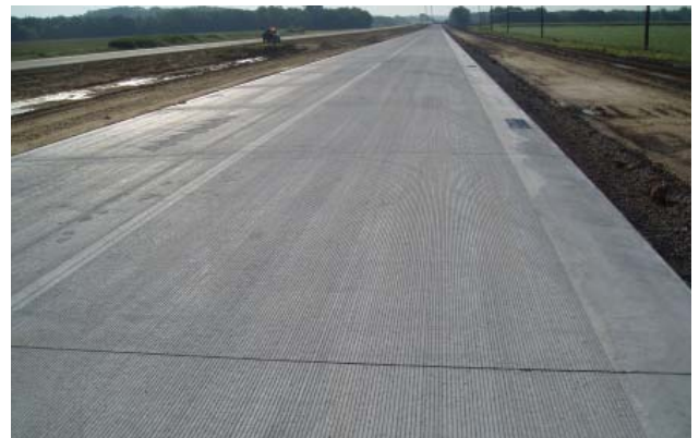
Longitudinal texture on concrete pavement
