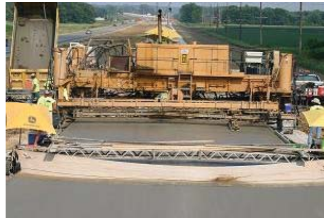
Burlap drag attached to paver
