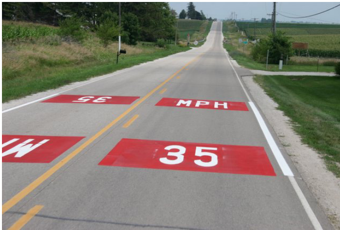
Figure 2. Example of pavement markings (surface treatment) (Hallmark et al./Institute for Transportation)
