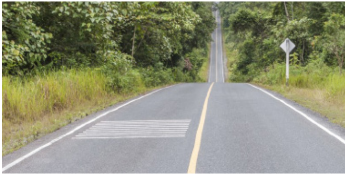
Figure 4. Advance stop line rumble strips (Shutterstock 2014)
