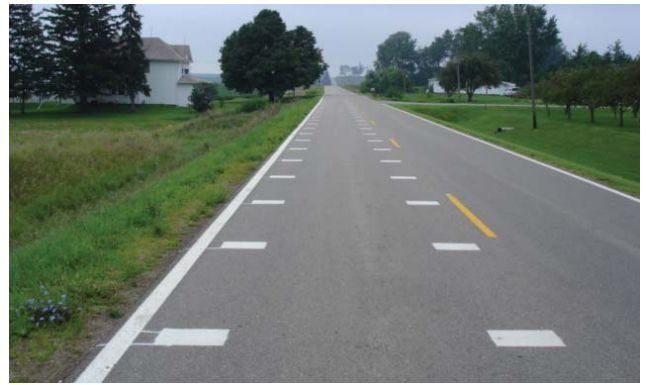
Peripheral transverse pavement markings
