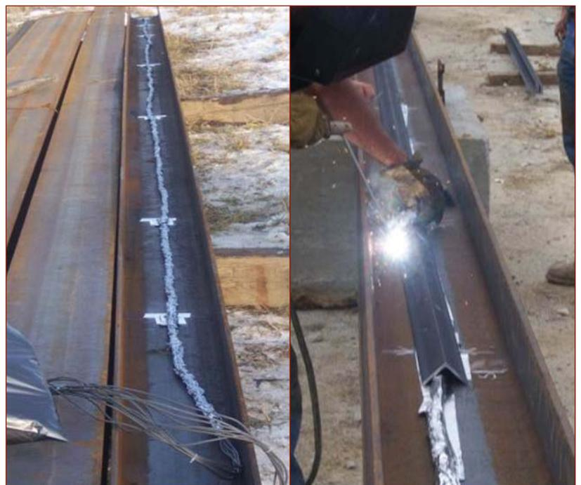
*Pile instrumentation (left) and its protection (right)*
