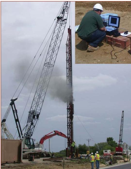
Pile installation with restrikes and PDA (inset)
