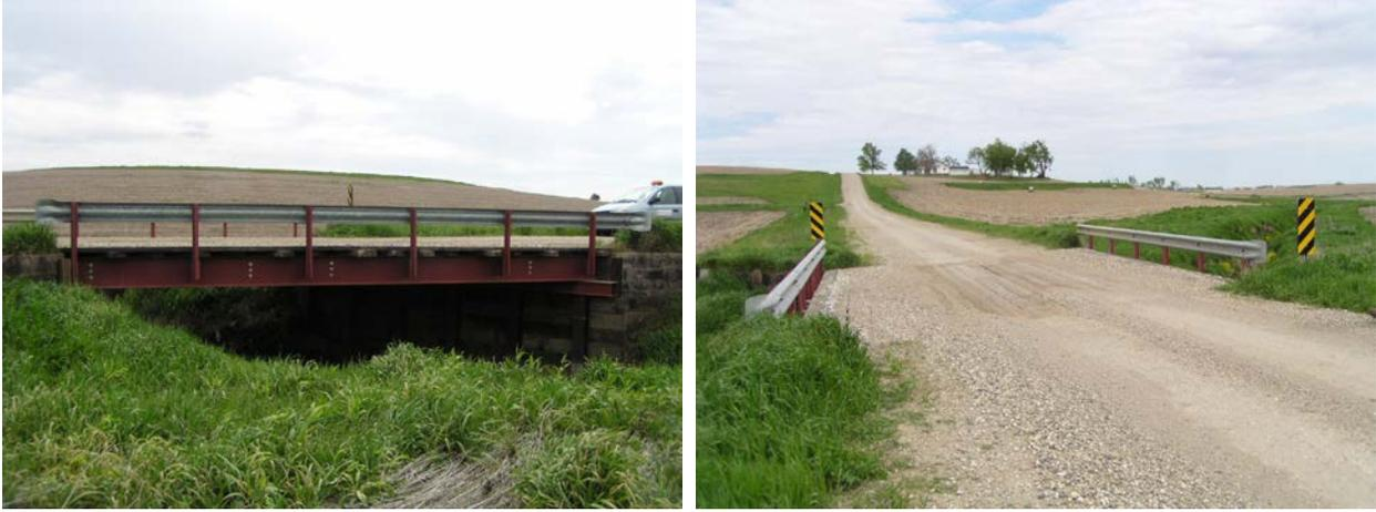
**Figure B-10. Steel-Timber Bridge 2: South elevation view (left) and west end view (right)**
