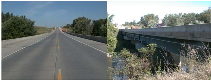
FIGURE 1. Photographs of Bridge Deck and Profile
