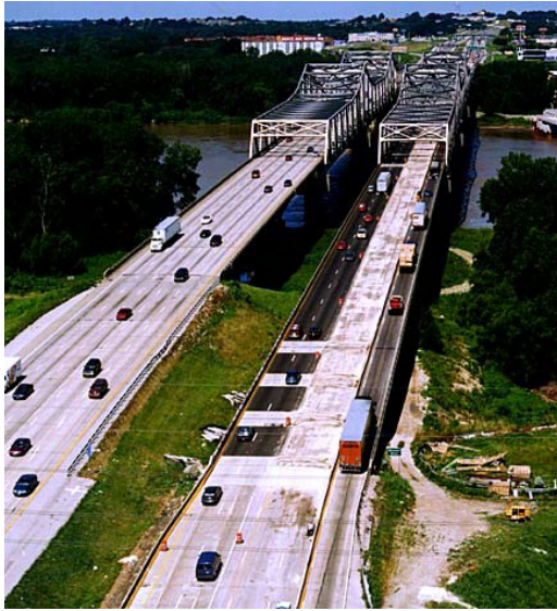
Construction on Blanchette Bridge in St. Louis, Missouri
