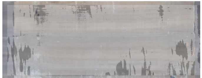
Infrared thermal imaging results for the entire Mud Creek Bridge deck
