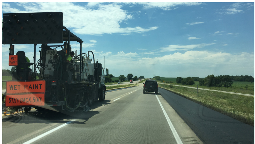
Rear view of pavement marking operation on interstate highway in Iowa
