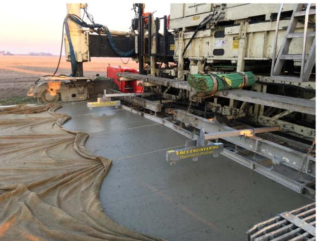
Create a slot of sufficient width in the drag underneath the RTS sensors.
