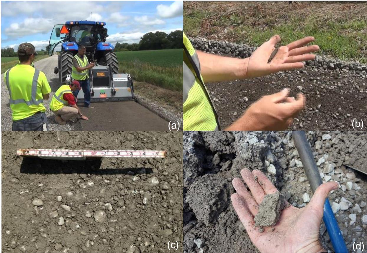
**Figure 4.23. Construction of Test Section 3: (a) mixing Virgin Aggregate 2 with existing surface material using FAE reclaimer, (b) checking plasticity of fine particles, (c) the new surface material after compaction, and (d) Virgin Aggregate 2 of the stockpile in the quarry**
