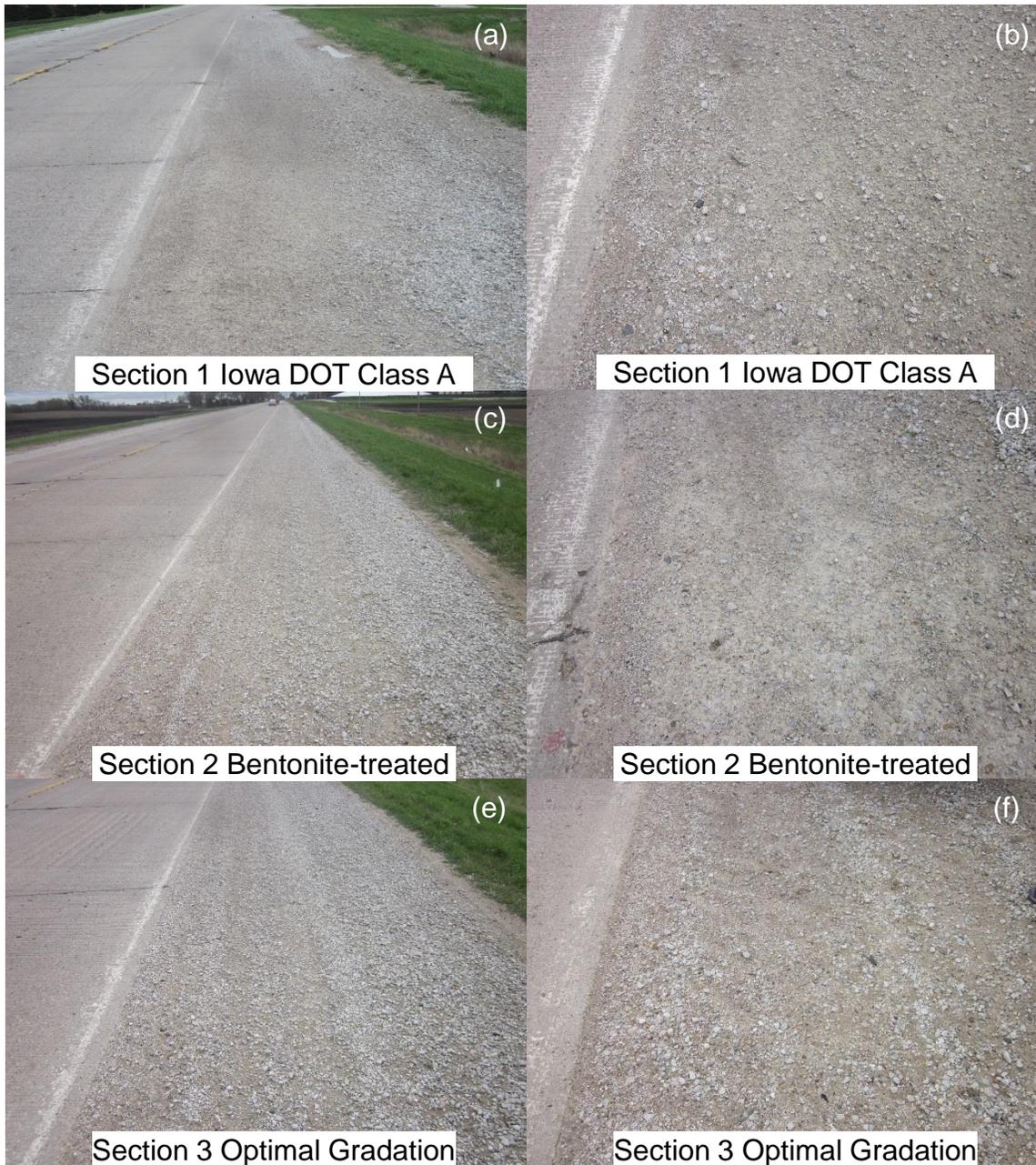
**Figure 4.46. Survey photos of T Ave. shoulder test sections taken on April 20, 2017**
