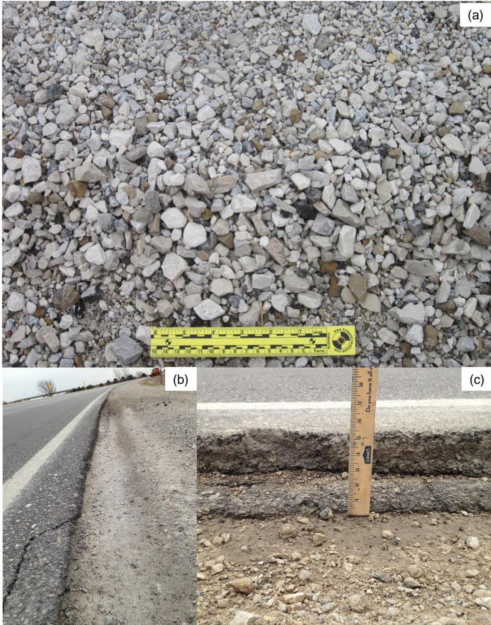
**Figure 4.15. Survey photos of Highway 30 ramp section (granular shoulder test Site 2): (a) surface material on November 3, 2015, (b and c) edge drop-off on March 22, 2016**
