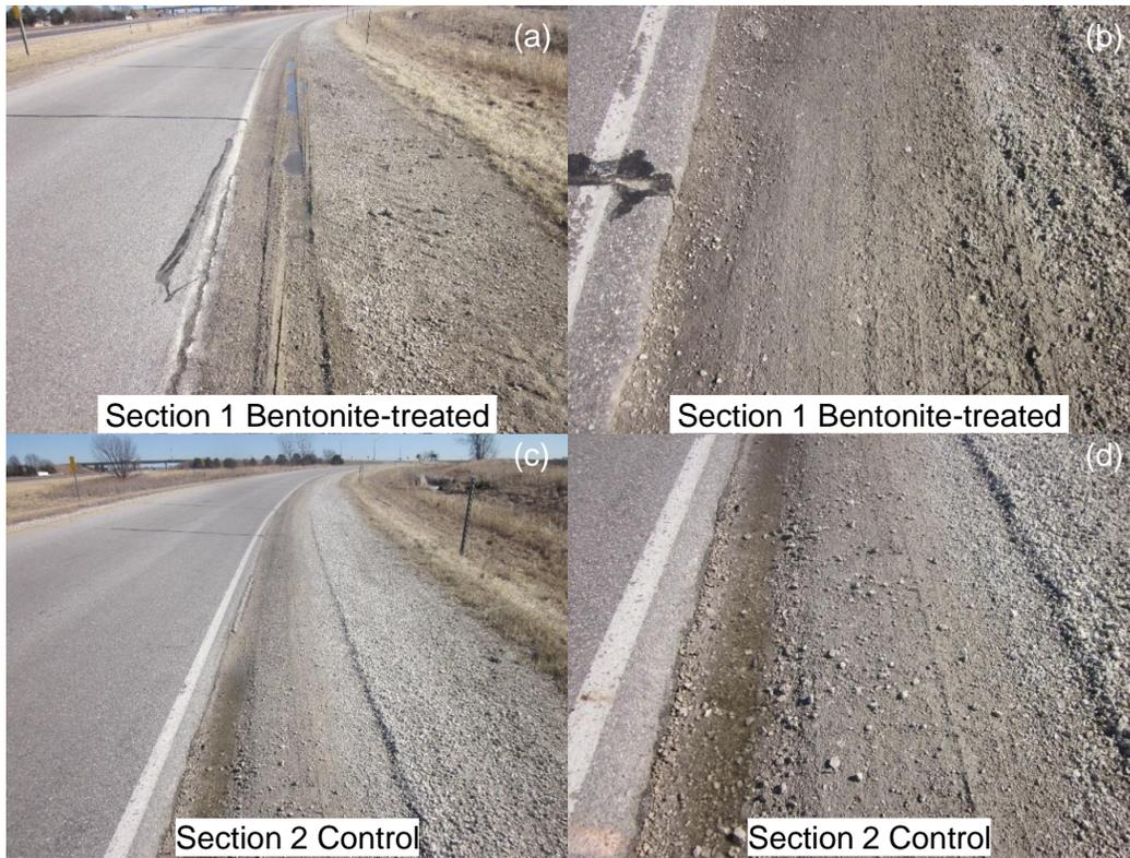
**Figure 4.54. Survey photos of Hwy 30 off-ramp shoulder sections from February 12, 2017**
