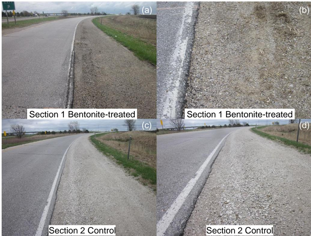
**Figure 4.55. Survey photos of Hwy 30 off-ramp shoulder sections from April 20, 2017**
