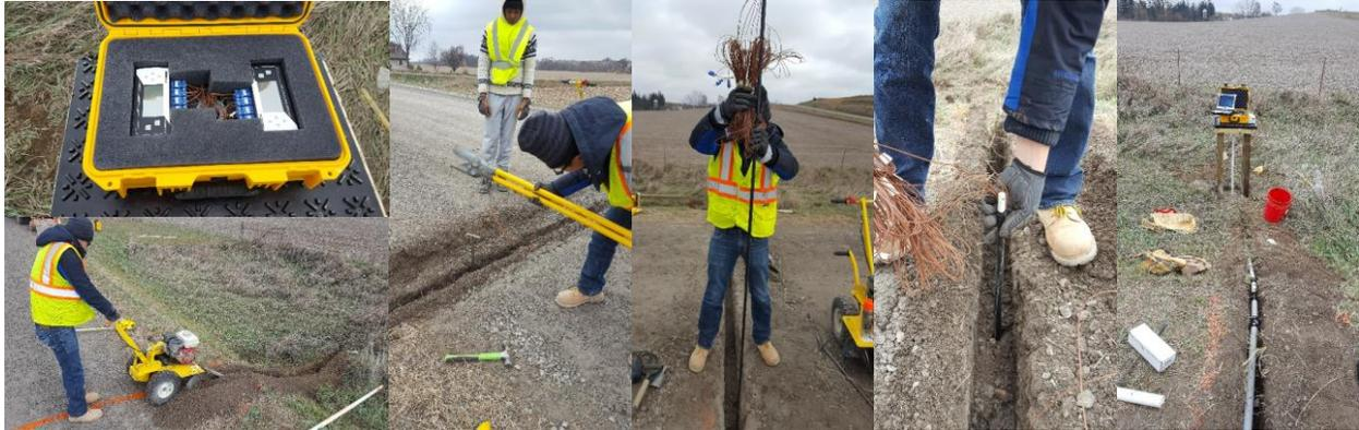
**Figure 4.10. Installation procedure for the subgrade temperature sensors**
