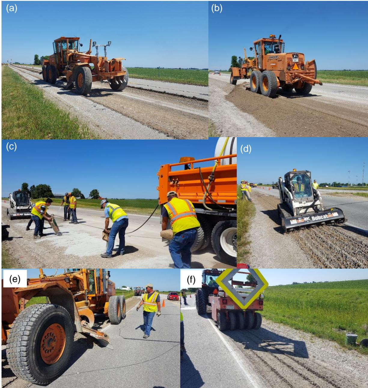
**Figure 4.28. Construction procedures of granular-surfaced shoulder test sections: (a) removing existing T Ave. shoulder surface material with a motor grader, (b) mixing virgin and existing material on road surface and placing back on the shoulder, (c) spreading bentonite powder on surface of Section 2 and spraying with water, (d) incorporating bentonite with a soil tiller, (e) shaping the treated material with a motor grader, and (f) compacting using a rubber tire roller**
