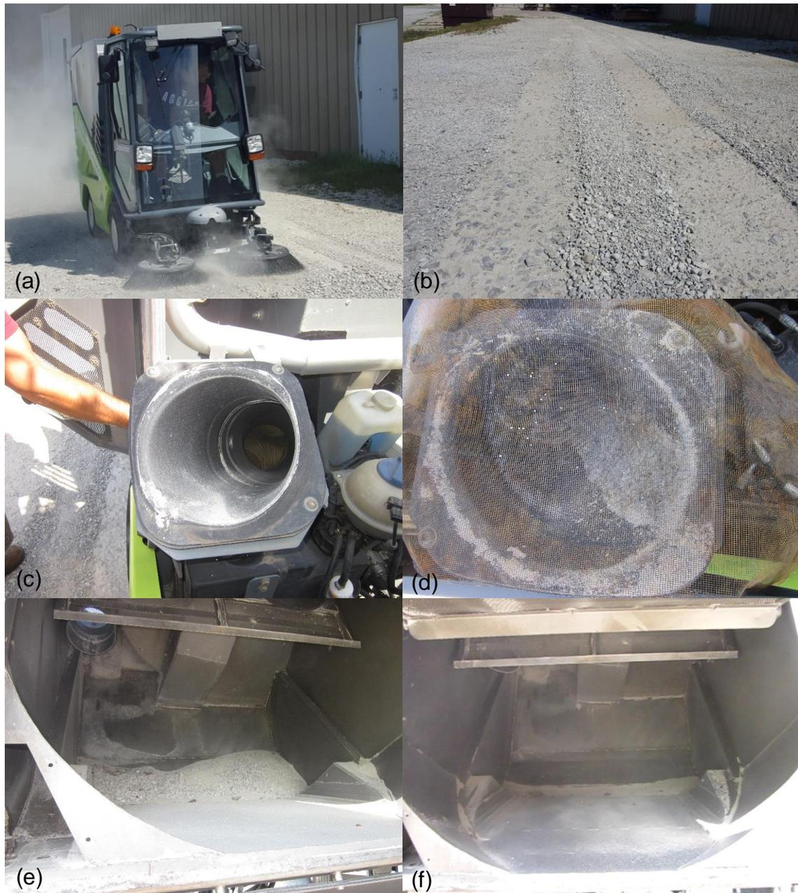
**Figure 4.18. Demonstration of using a vacuum street sweeper to remove fines of granular surface materials: (a) vacuum street sweeper, (b) vacuumed roadway surface with coarse material brushed to center and sides, (c) vacuum chute without a screen, (d) vacuum chute with screen installed to retain coarse material on road, (e) material in the hopper vacuumed without the screen, and (f) material in the hopper vacuumed with a screen**
