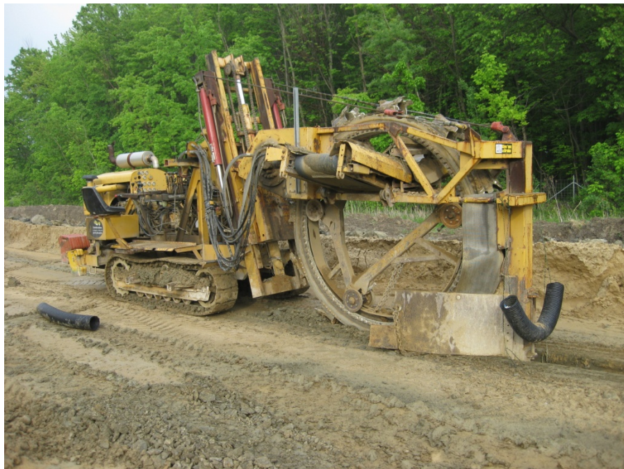
Figure 6. Subgrade layer after undercutting (top) and trench drain installer (bottom)
