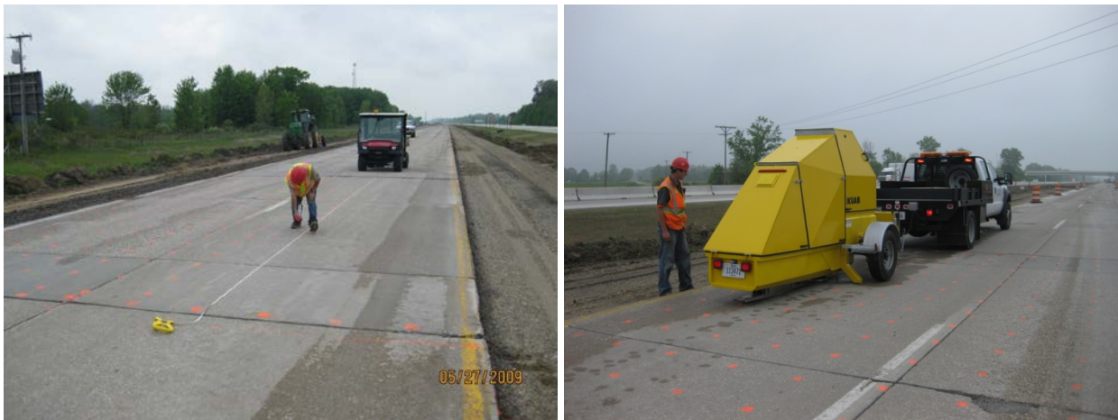
Figure 71. TS2-B: Laying out the test grid (left) and Kuab FWD testing on the grid (right)
