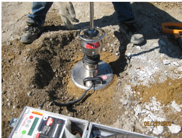
Figure 77. TS2-B: Plate load testing in progress
