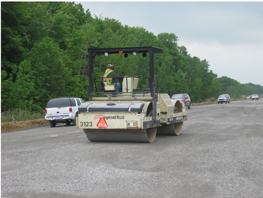
Figure 8. OGDC base layer placement and compaction
