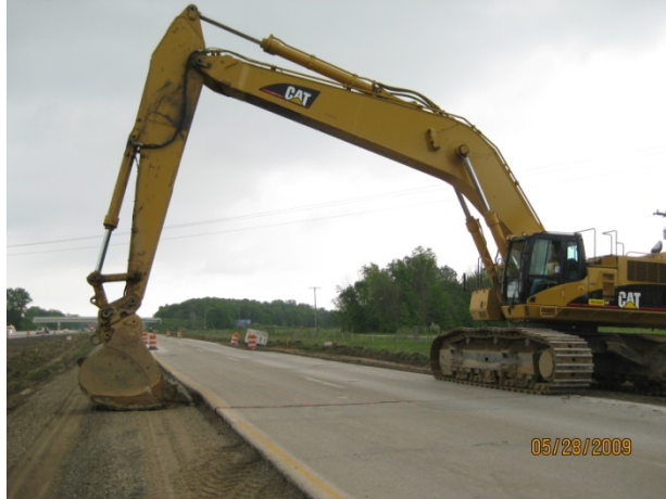
Figure 72. TS2-B: Bucket loader in place for excavating existing pavement
