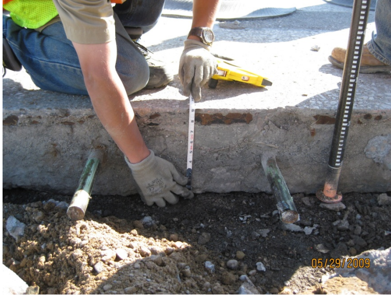
Figure 2. Thickness of the existing PCC pavement and existing foundation material
