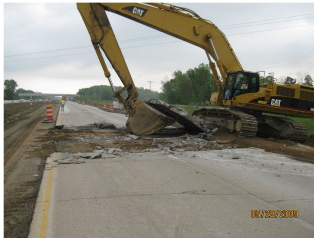
Figure 73. TS2-B: Bucket loader excavating existing pavement
