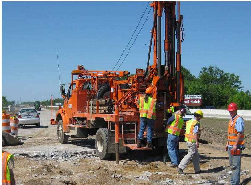
Figure 12. MDOT drill rig used to obtain Shelby tube samples from subgrade
