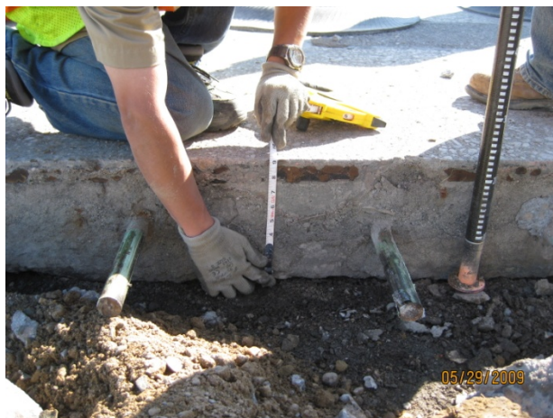
Figure 74. Measuring the existing pavement depth
