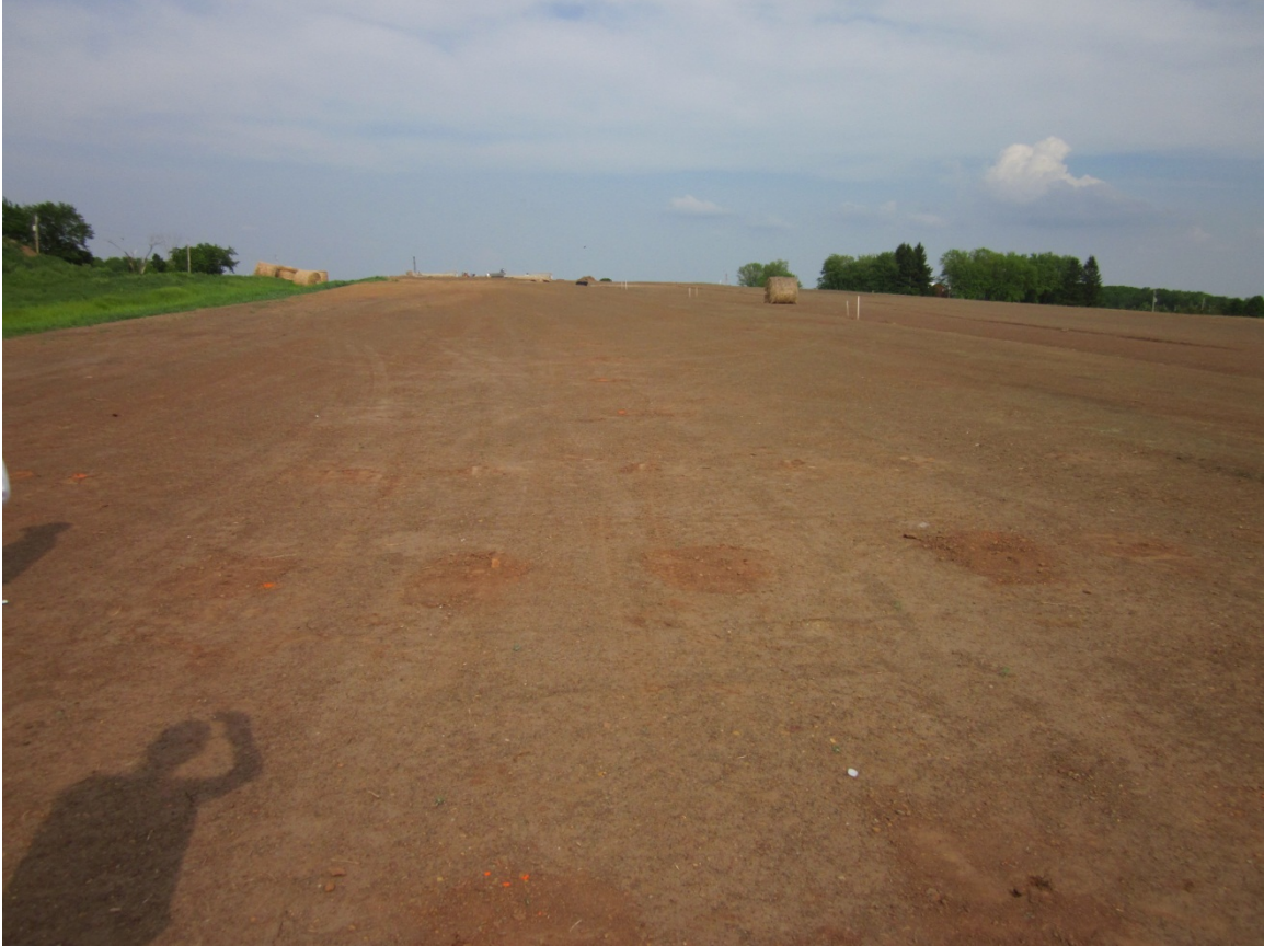
Figure 41. TS2: Photograph of the compacted subgrade
