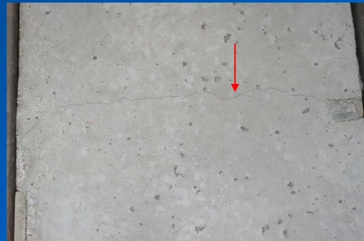
Cracked Slab
