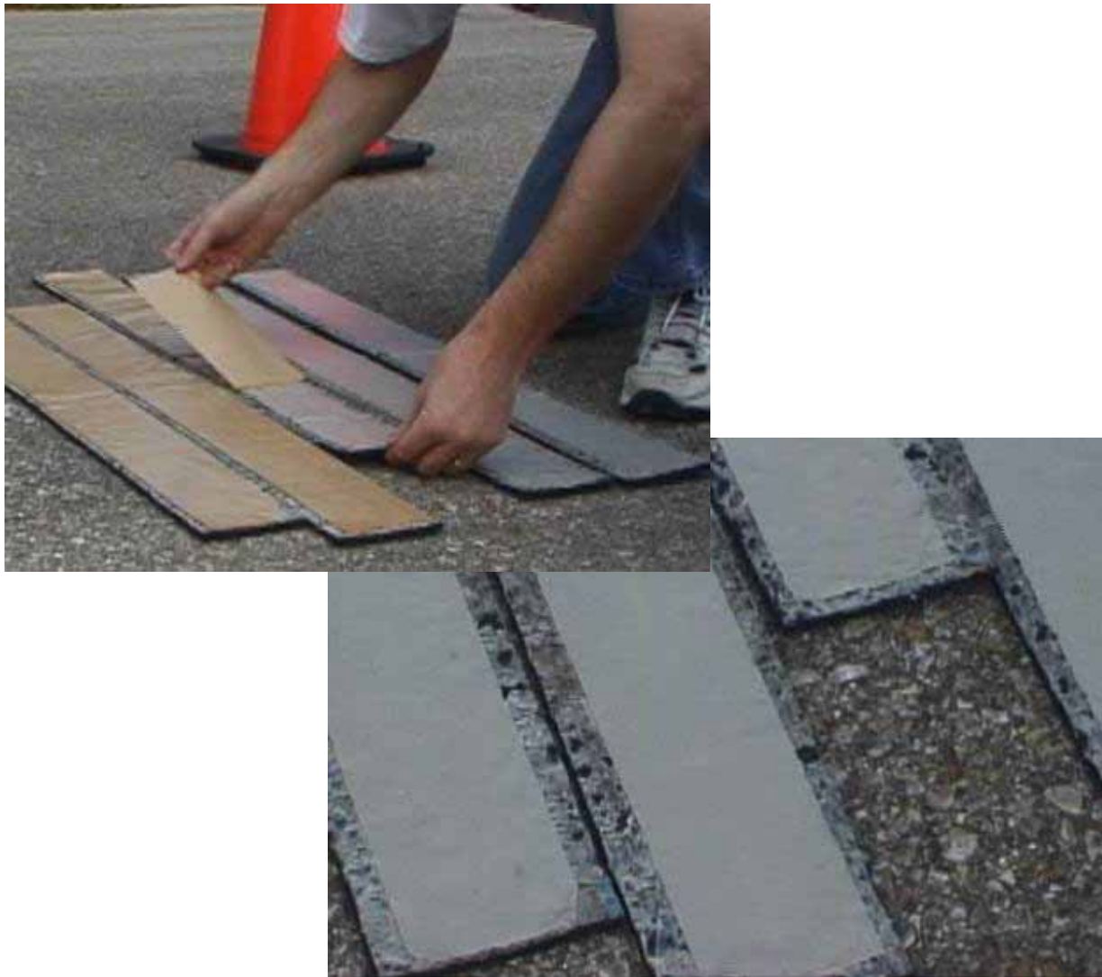
Figure 2. Applying replacement adhesive.
