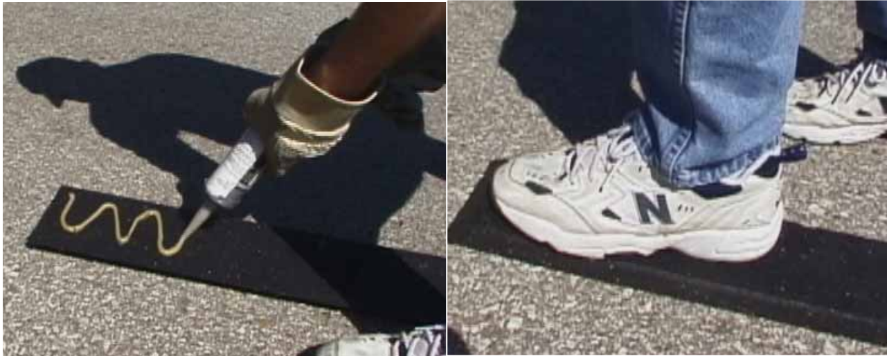
Figure 1. Applying urethane adhesive (left) and applying pressure to the strip (right).
