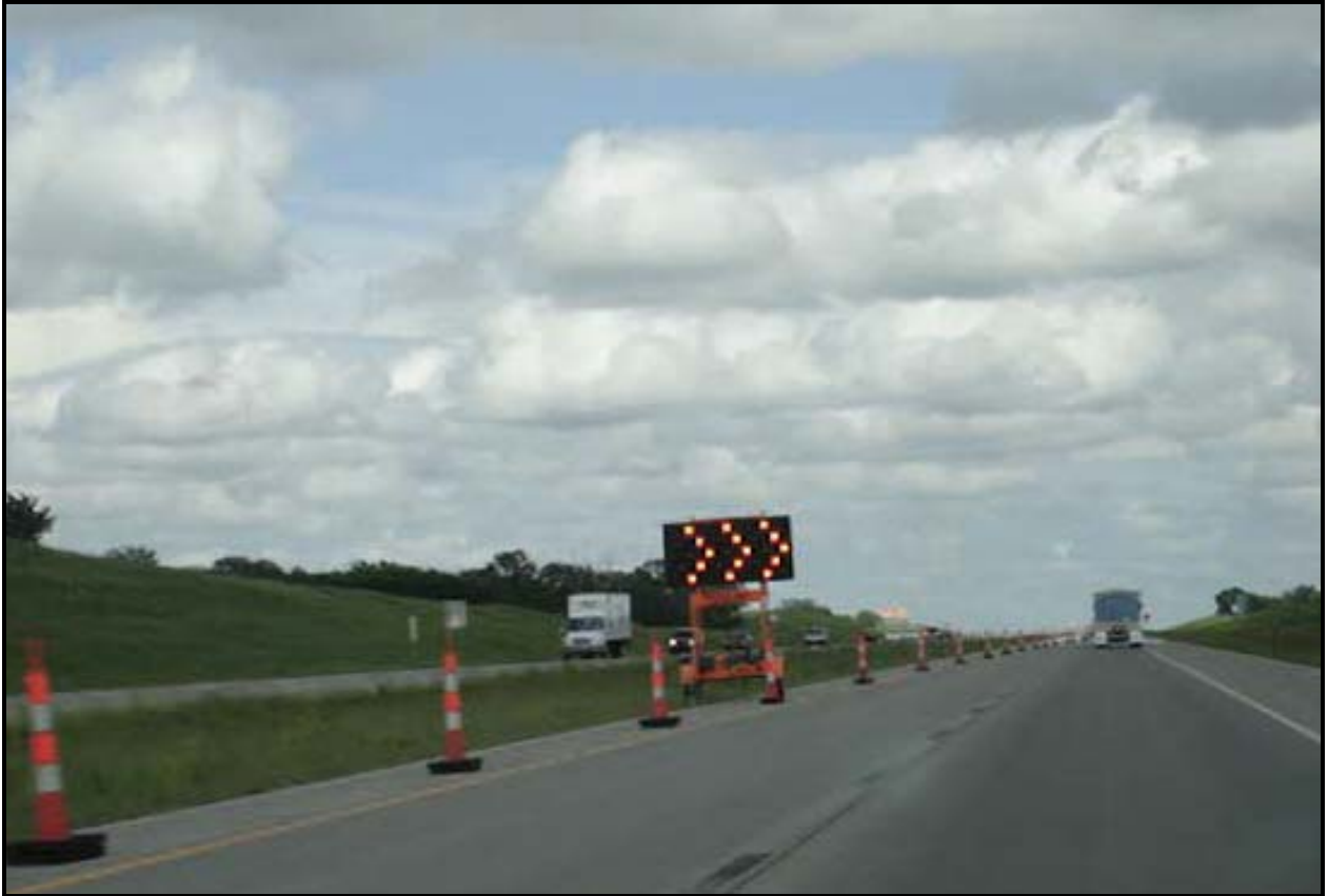
FIGURE 2 Typical advance warning arrow display at a long-term work zone (chevron displayed).
