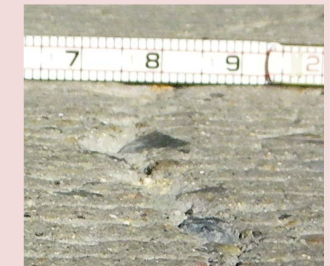
Wide cracks with spalled edges
