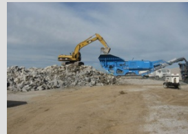
Loading the Crusher
