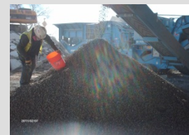
Inspector Removing Debris
