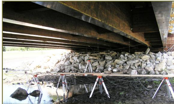
**Completed FRP reinforced glulam girder bridge with condition monitoring sensors attached.**
