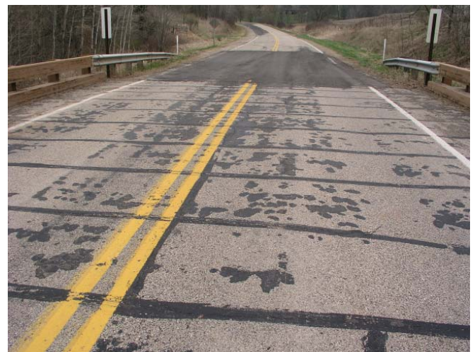
Figure 11. Erfurth Bridge wearing surface.
