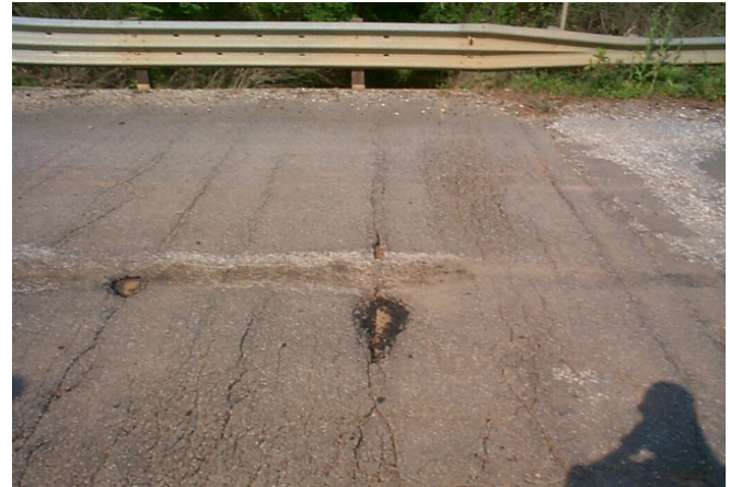
Figure 3. Chambers County Bridge wearing surface.
