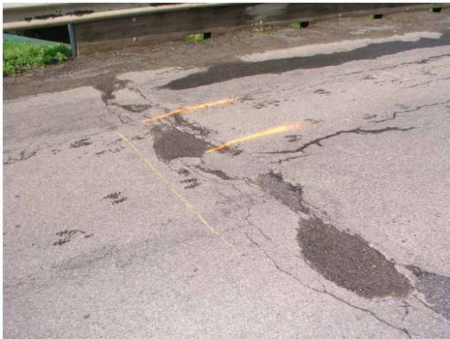
Figure 18. Bolivar Bridge 2003 entrance abutment.
