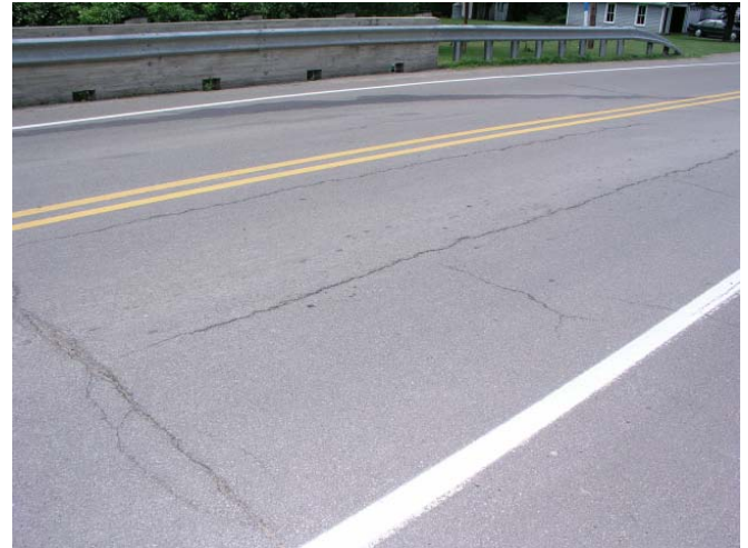
Figure 16. East Main Street Bridge 2003 asphalt wearing surface.
