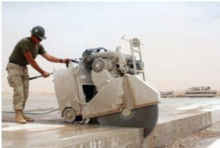
The time of sawing is critical to prevent raveling or cracking. The newly poured concrete for the paving application must develop enough strength to allow saw equipment to get on the slab. Sawing must be completed before the concrete has developed too much strength, leading to the development of random cracks. A calorimetry test measures the heat release in concrete, thereby determining the degree of hydration,
