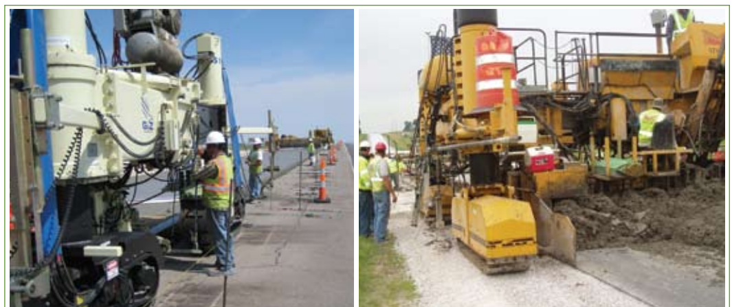
Figure 1: Stringline (left) and stringless (right) pavers
