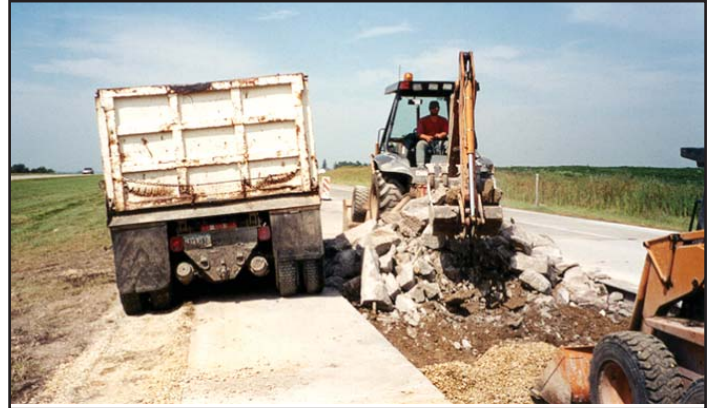
Figure 6. Concrete removal using a backhoe
