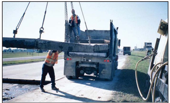
Figure 7. Concrete removal using the lift-out method
