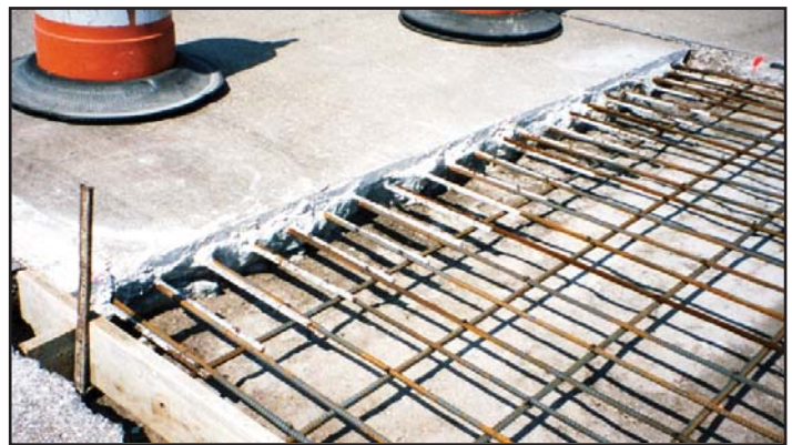
Figure 11. Example of CRCP FDR
