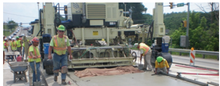
Placement of 6-in. bonded concrete overlay on SR-119, Pennsylvania
