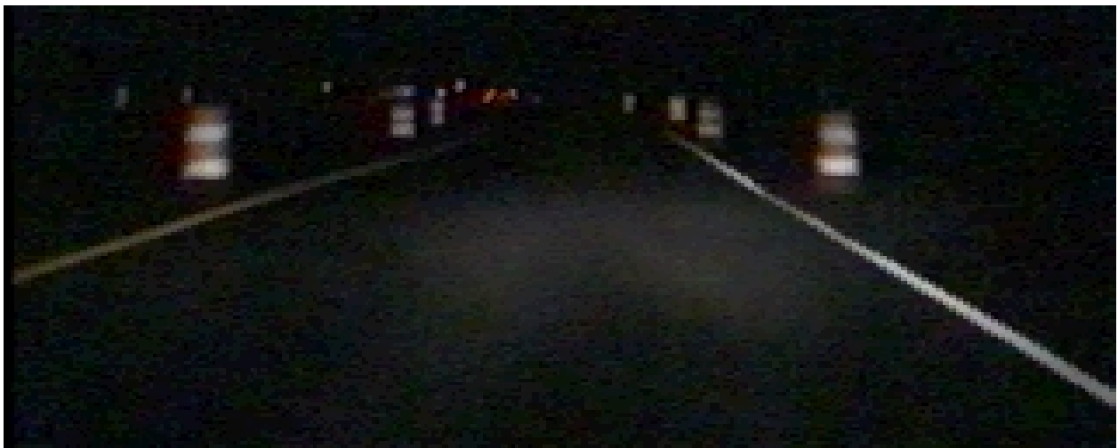
FIGURE 3-8 Crossover without lighted delineation.
