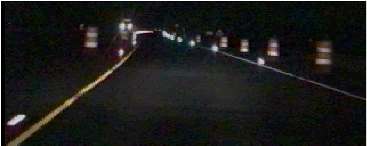
FIGURE 3-7 Crossover delineated by Lightguard Lighted RPMs.
