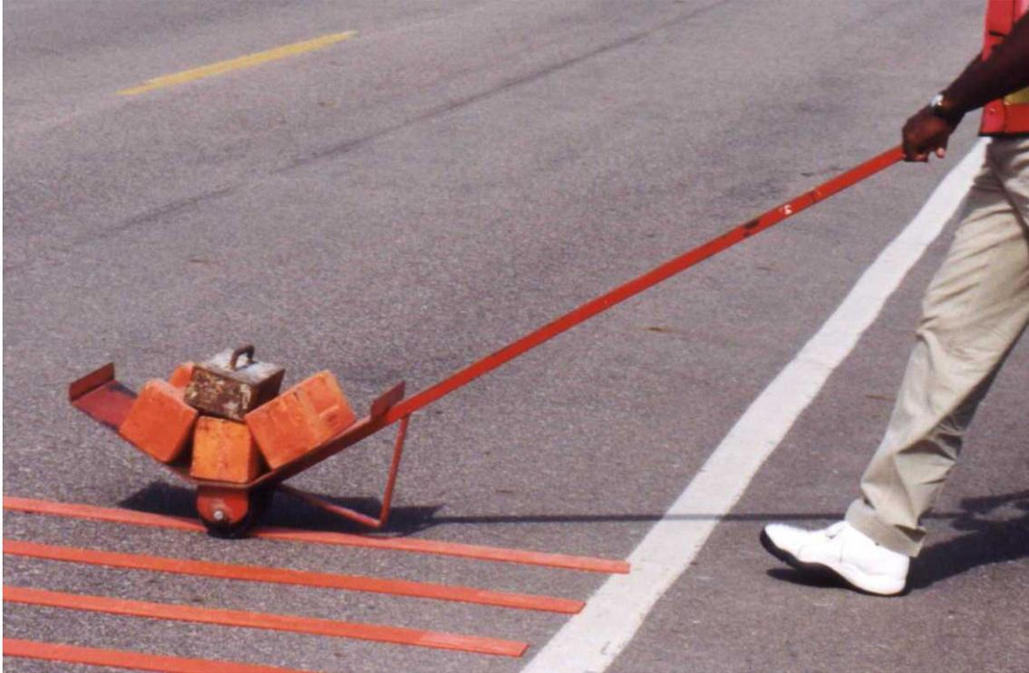
**Figure 5. Tampering Card Used During Installation**
