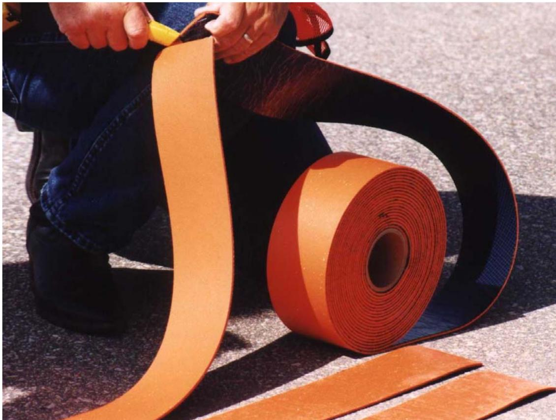
**Figure 4. Cutting Rumble Strips to Appropriate Length**
