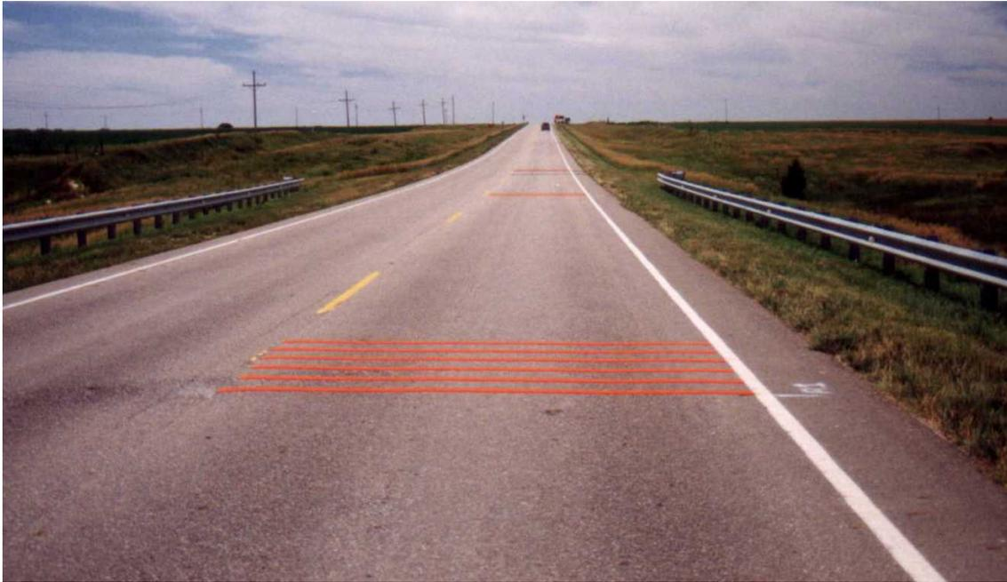
**Figure 3. Removable Rumble Strip Evaluation Installation**
