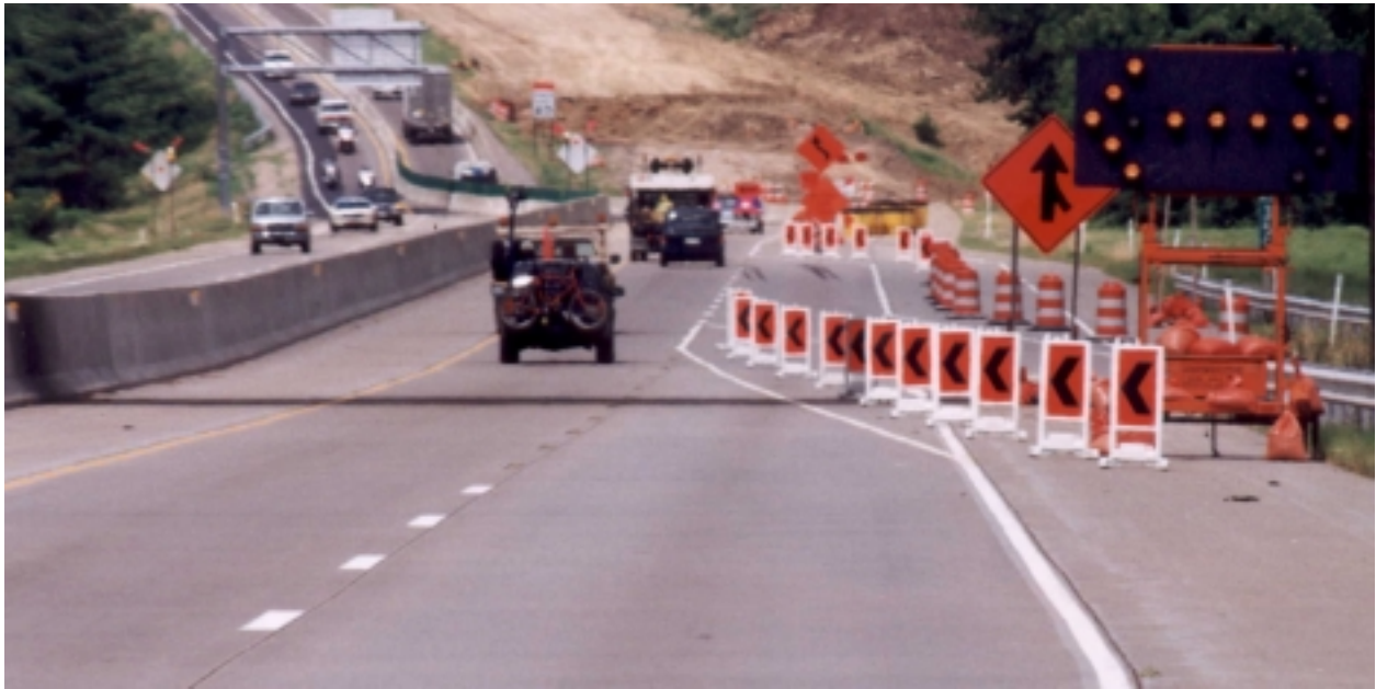
FIGURE 3-14 Vertical SafetyCade test site.
