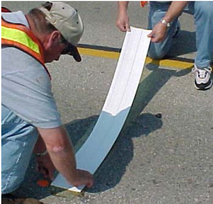
Figure 1. A Strip of the Rumbler Being Glued to a Road
