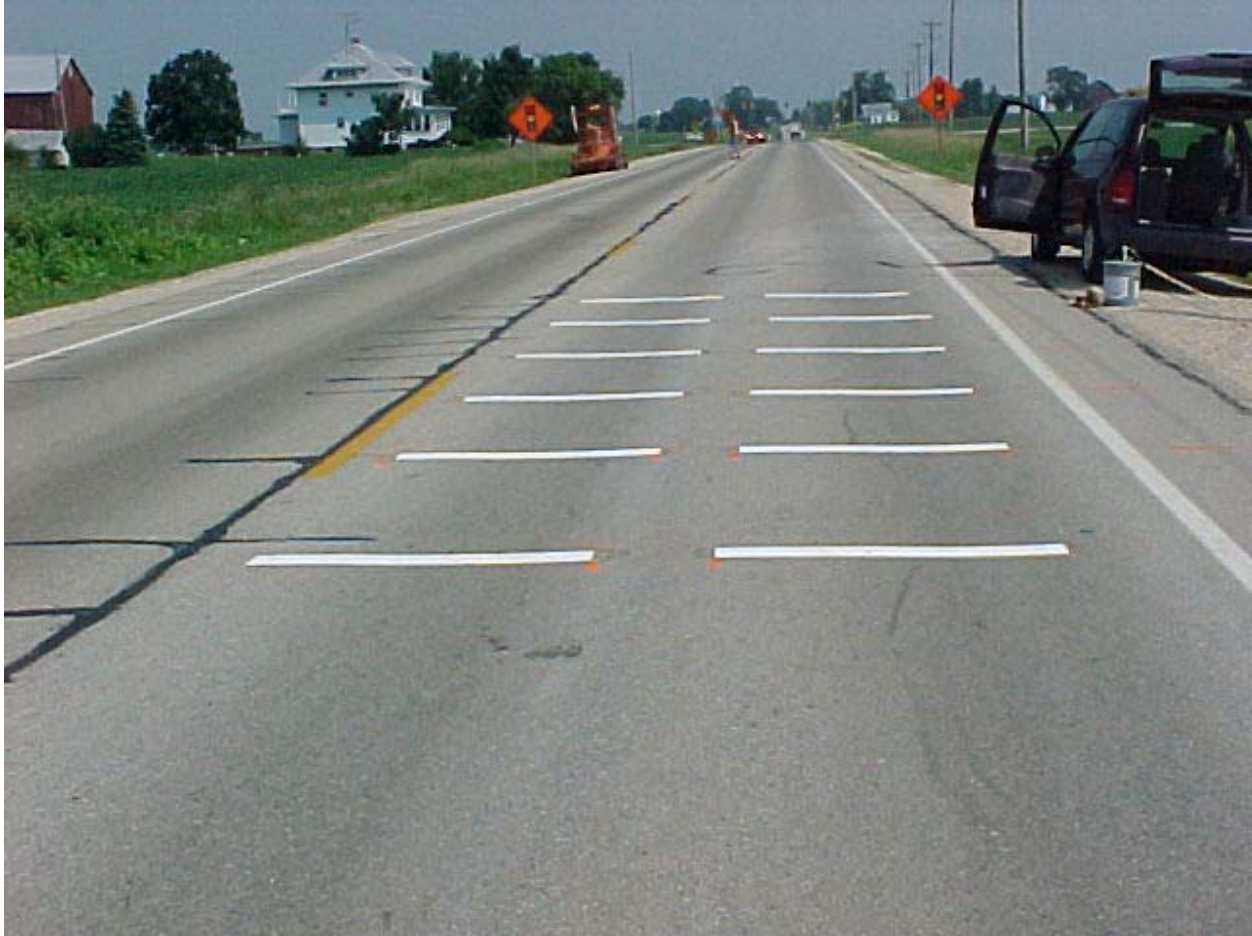
Figure 2. Rumbler as Installed on STH 26
