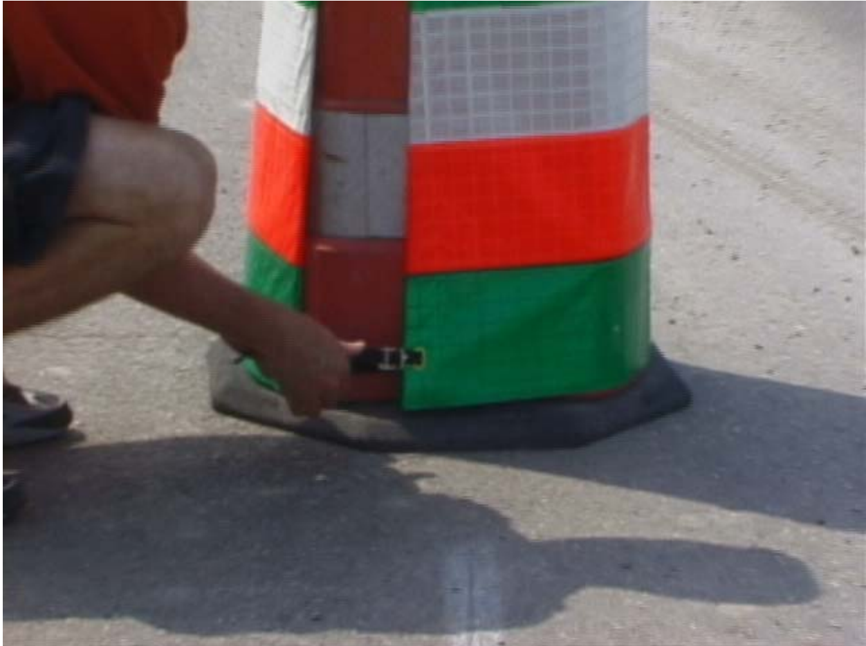
Figure 4. Drum sleeve installation.
