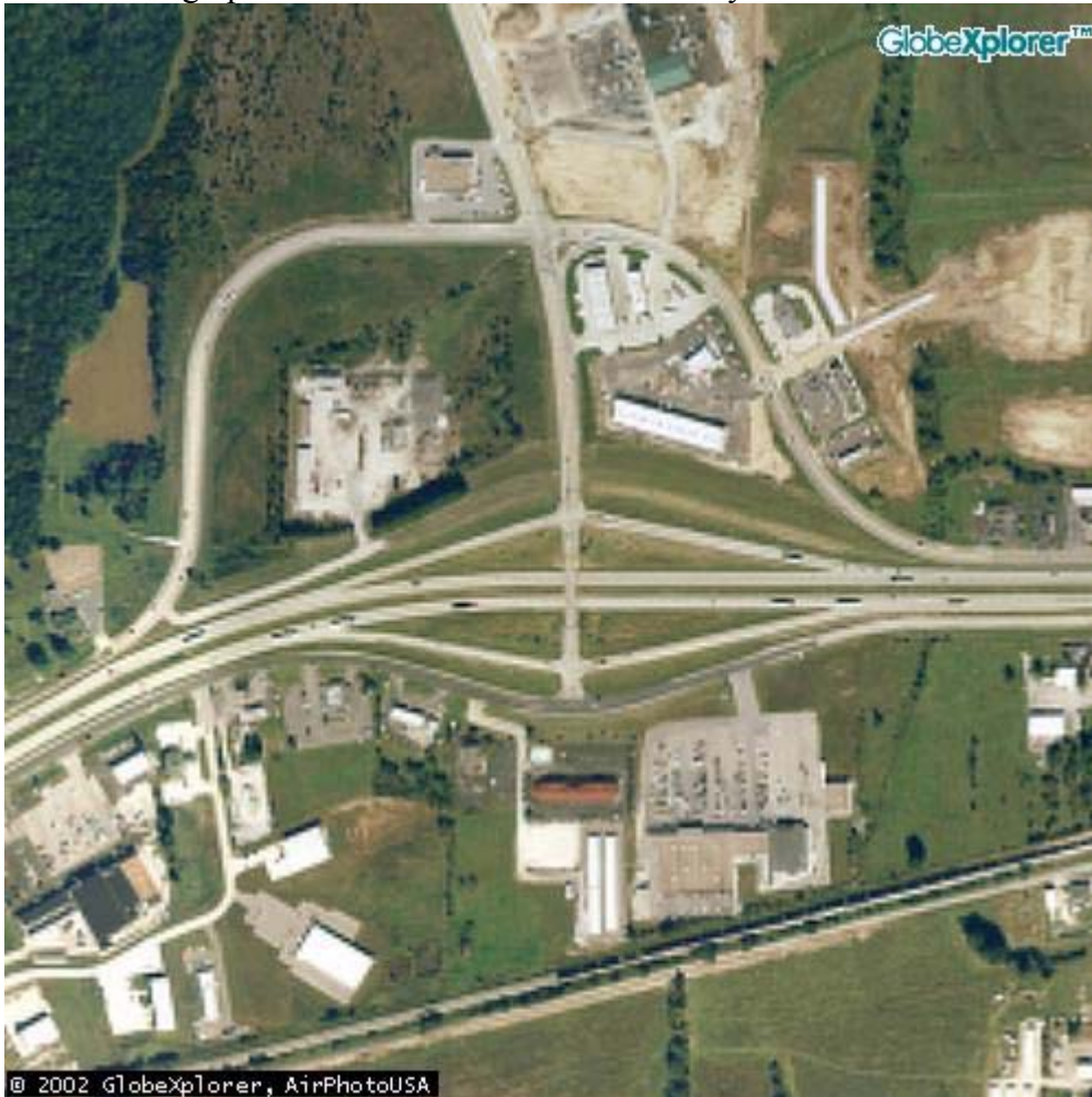
Aerial Photograph from the I-70 at Wentzville Study Site
