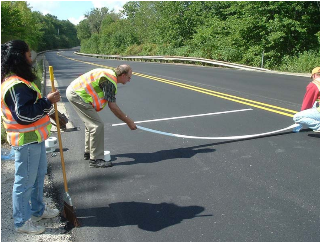
FIGURE 8 Installation of the Work Zone Test Rumble Strip
