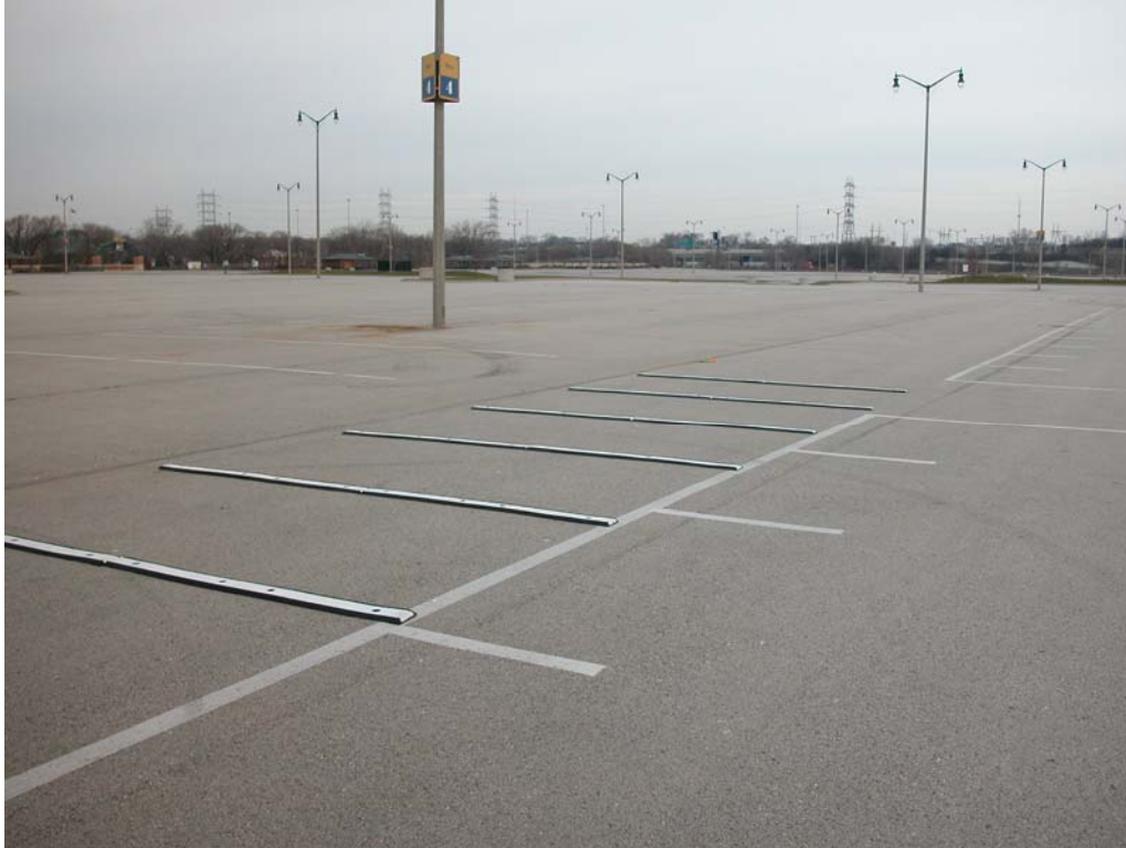
Figure 3 Deployment of RTI Bumps in Parking Lot at Seven Foot Spacing
