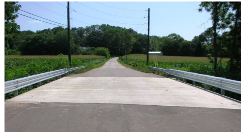
Internally cured bridge deck
