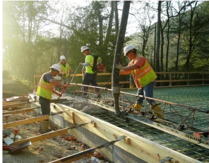
Plain concrete bridge deck was pumped
