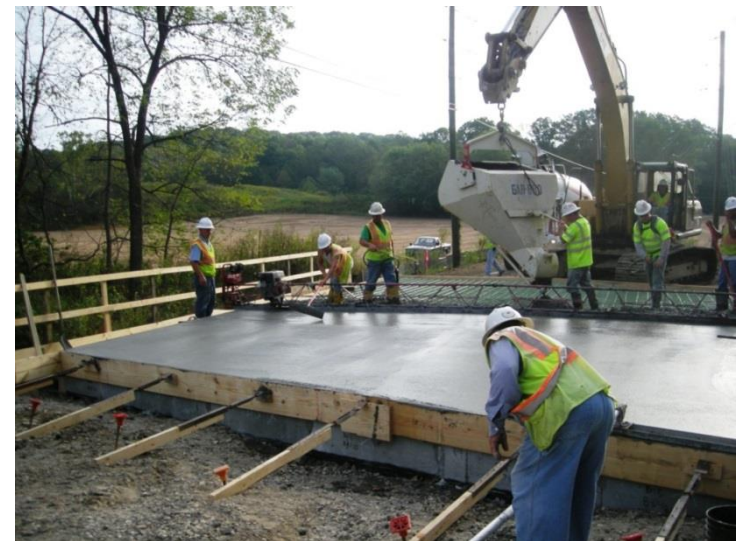
IC concrete bridge deck was placed by means of a bucket
