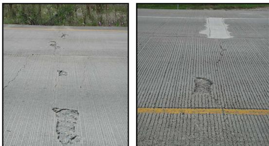
Figure 1: Typical Shallow Spalling in CRCP
