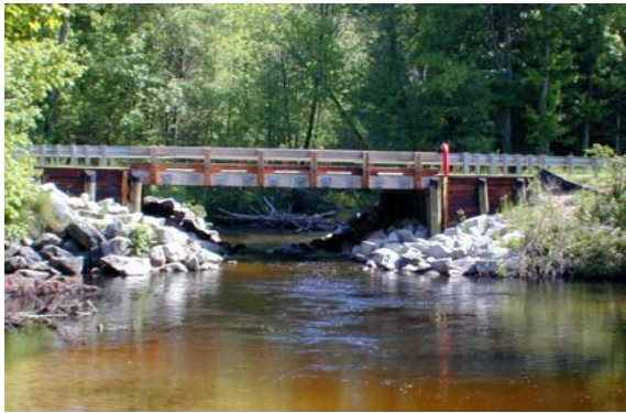
North Sharon Road Bridge
