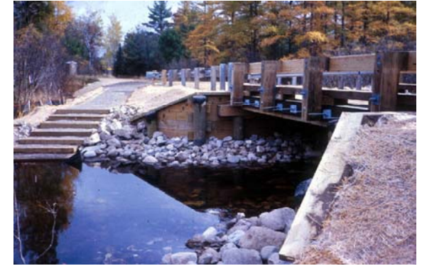
Lewiston Grade Road Bridge
