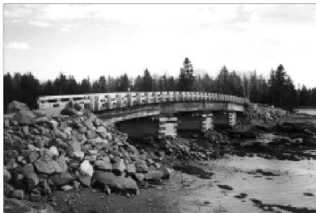
Crowley Island, Maine. 194 ft. long roadway bridge. Piers are wood and abutments are wood—eastern hemlock.
