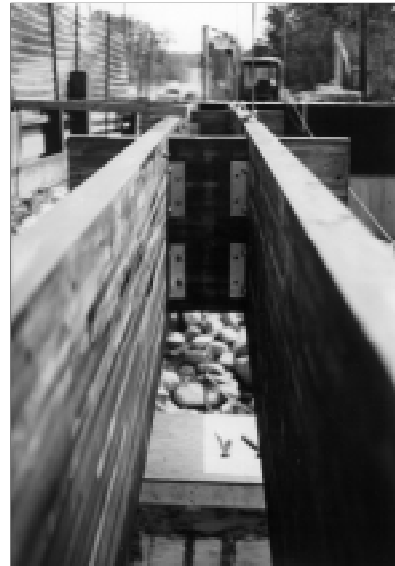
Construction of the Sangerville bridge utilizing all Maine red maple.
