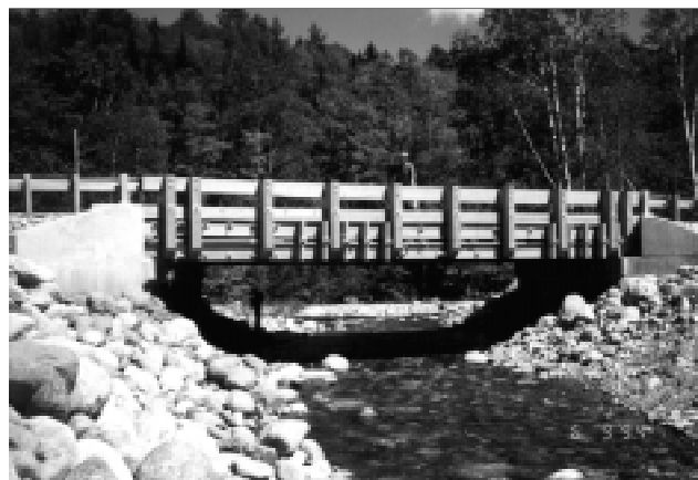
Completed Byron bridge.
