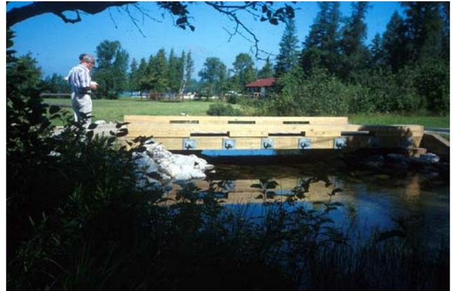
**Structure/Design Type:** Vehicular bridge/ Stress-laminated sawn lumber
