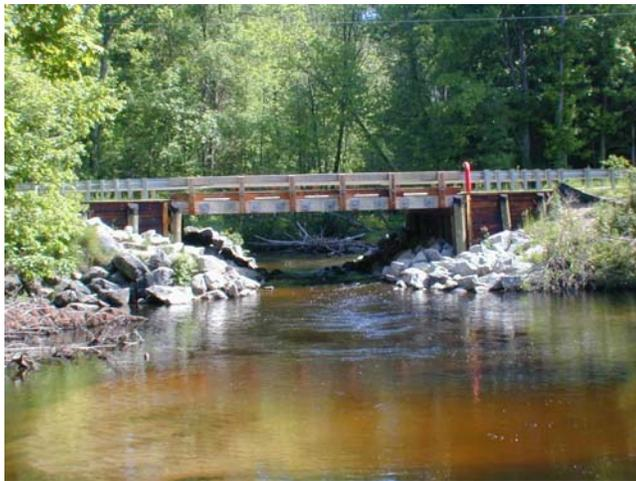
**Structure/Design Type:** Vehicular bridge/ Stress-laminated, glued laminated
