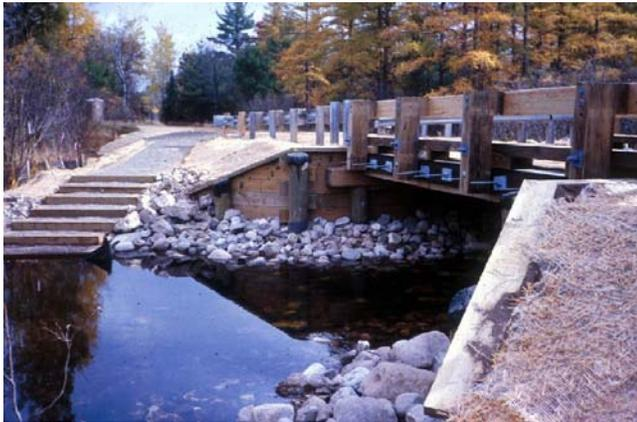
**Structure/Design Type:** Vehicular bridge/ Stress-laminated sawn lumber
