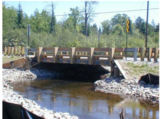
**Structure/Design Type:** Vehicular bridge/ Stress-laminated, glued laminated
