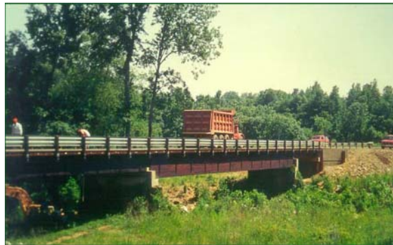
Glued laminated girder bridge.
