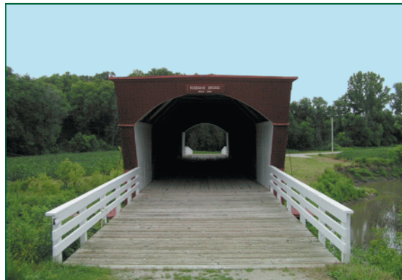
Roseman Bridge, Madison County, Iowa.
